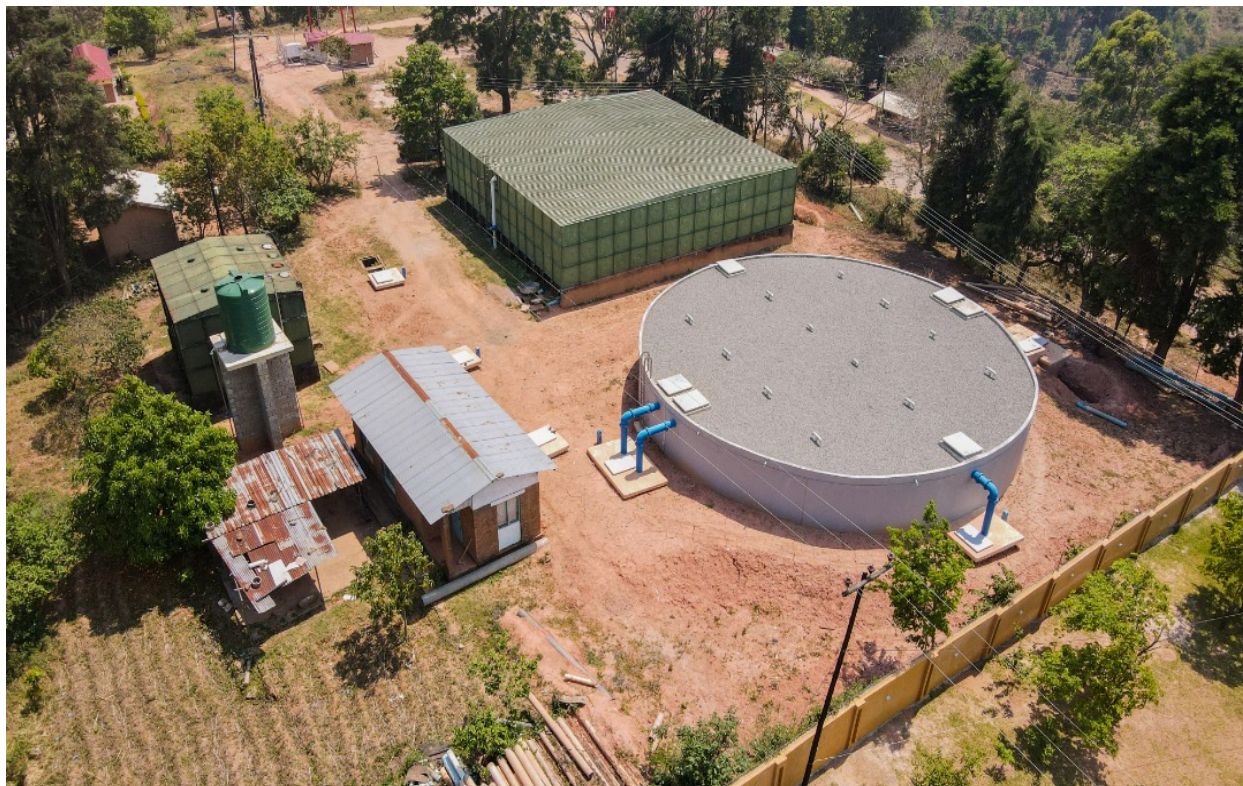
1,000 m 3 Signal Hill Concrete Tank - MZUZU
