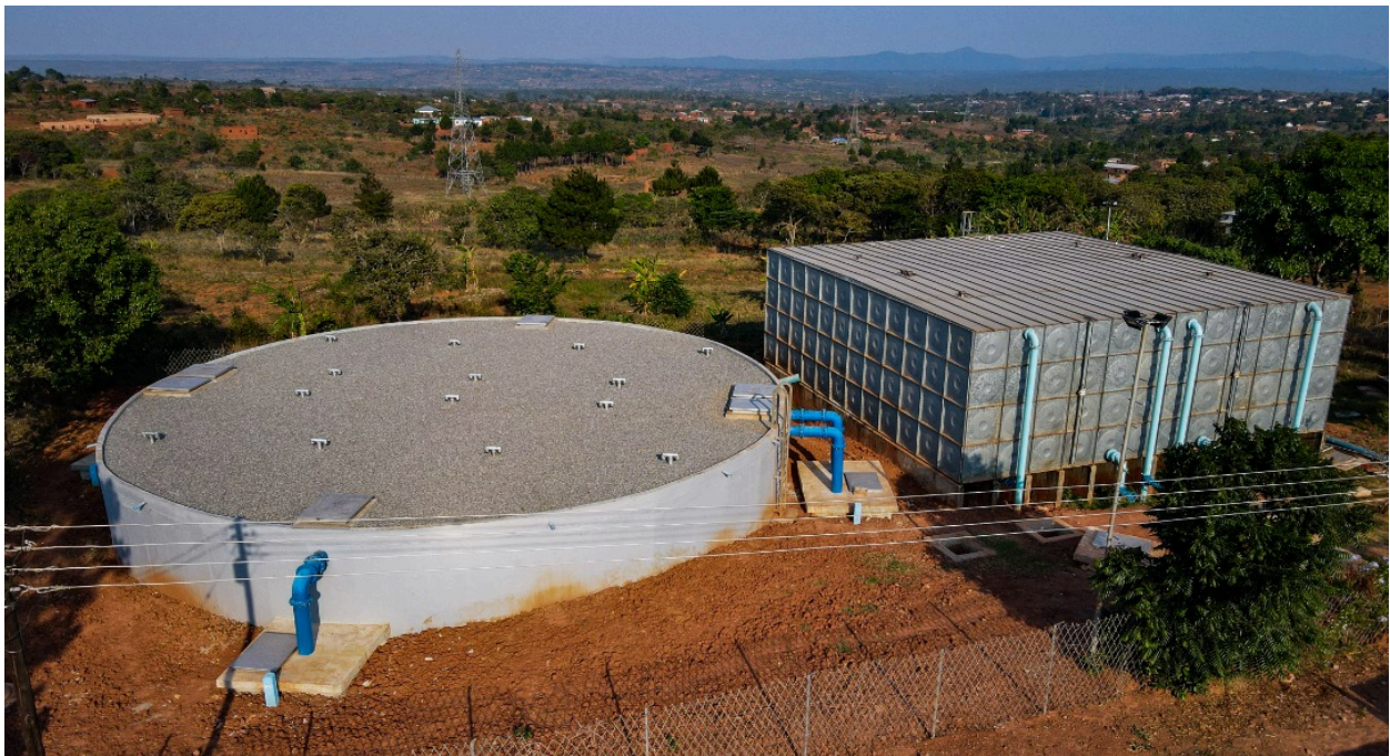
1,000 m 3 Nkhorongo Concrete Tank - Mzuzu
