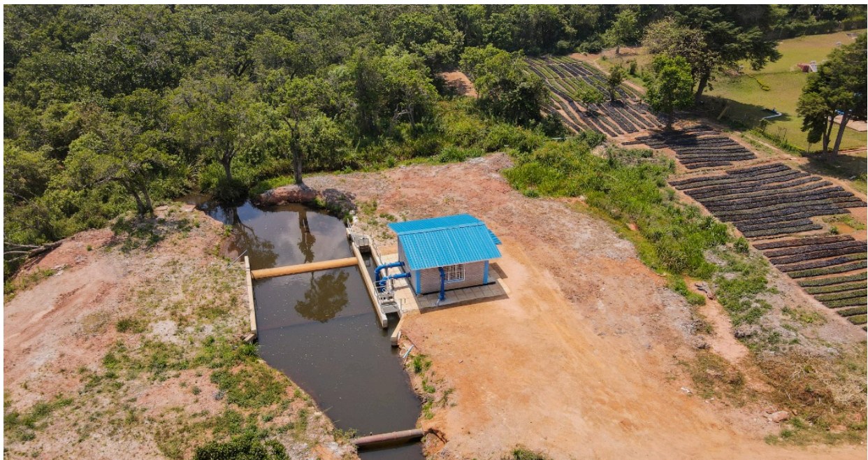
New Reinforced Concrete Weir downstream of Lunyangwa Dam at Mzuzu Treatment Plant completed in May 2021
