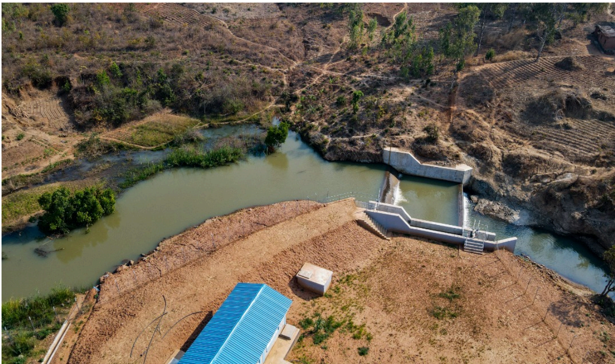
New Reinforced Concrete Weir at Ekwendeni Treatment Plant
