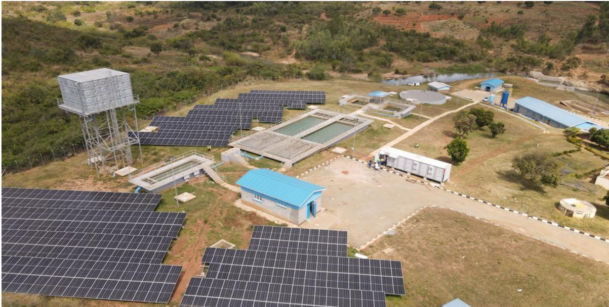
New 6,600 m 3 /day Ekwendeni Treatment Plant completed in February 2021 and Hybrid Solar PV System with Solar capacity 300 kWp & BESS Capacity 1,330 kWh completed in August 2022.
