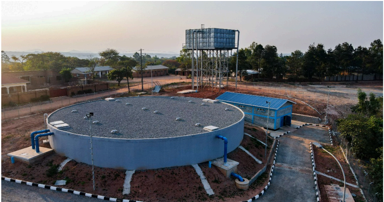
New 2,000 m 3 Reinforced Concrete Tank, 375 m 3 Elevated Tank and pump house at Lusangazi in Mzuzu
