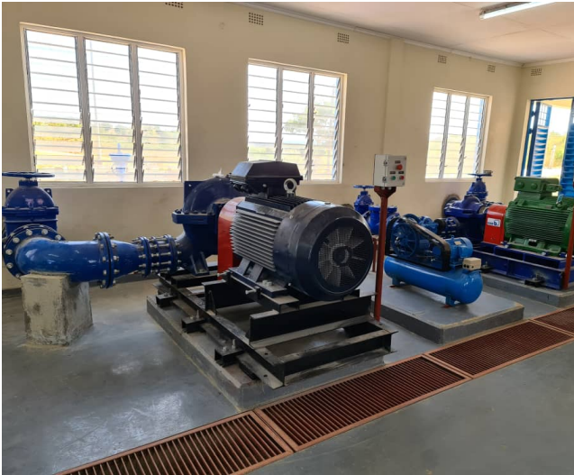
Pumps and pipework at Ekwendeni Treatment Plant
