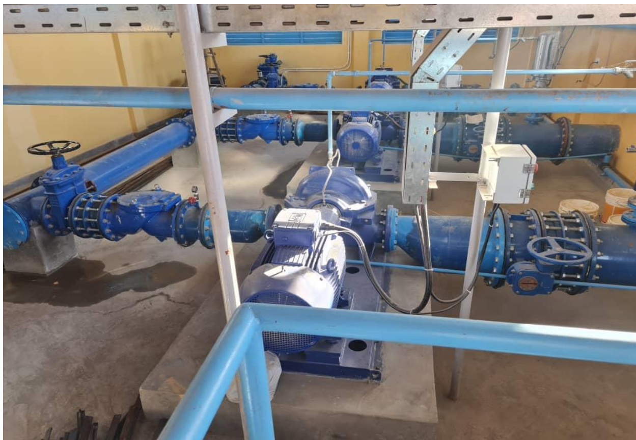
Water Treatment Plant - Raw Water Pumps
