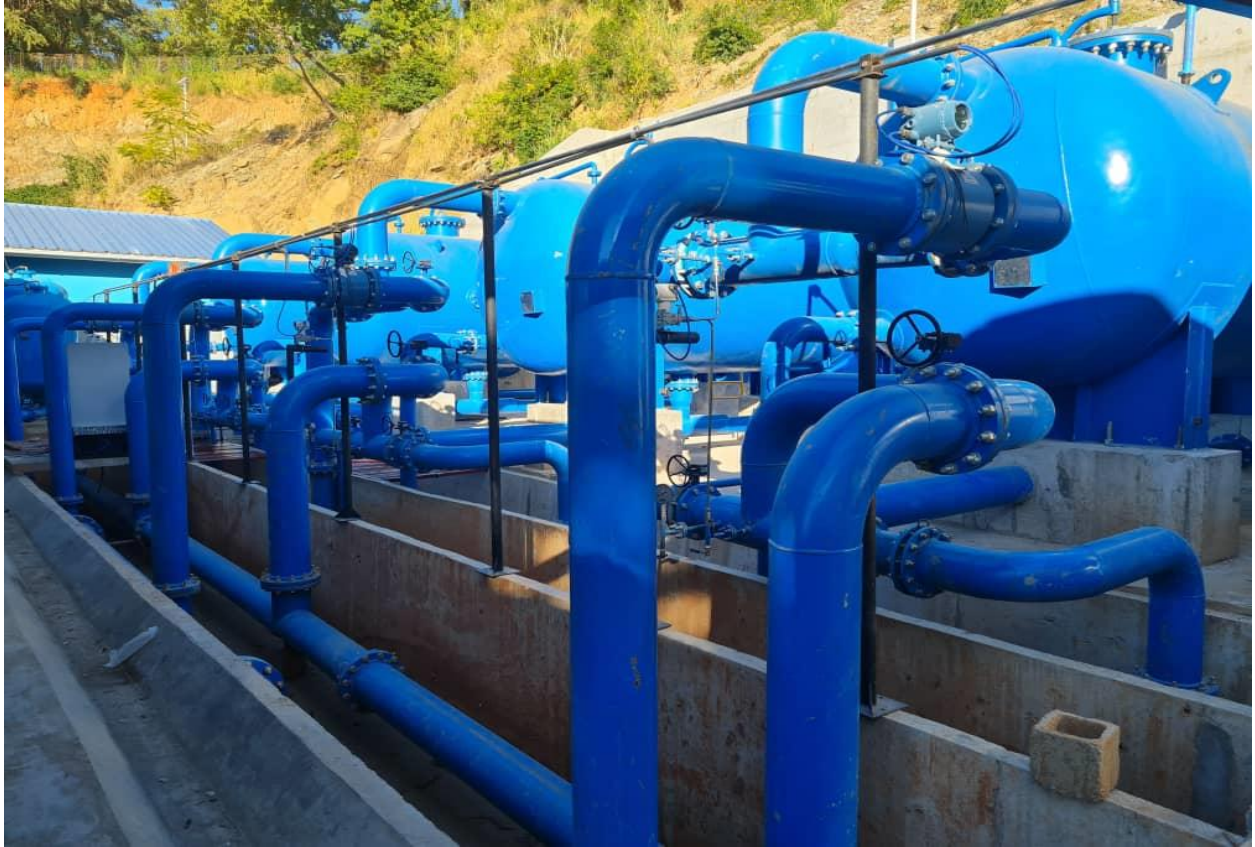
Water Pressure Filters at the Treatment Plant.
