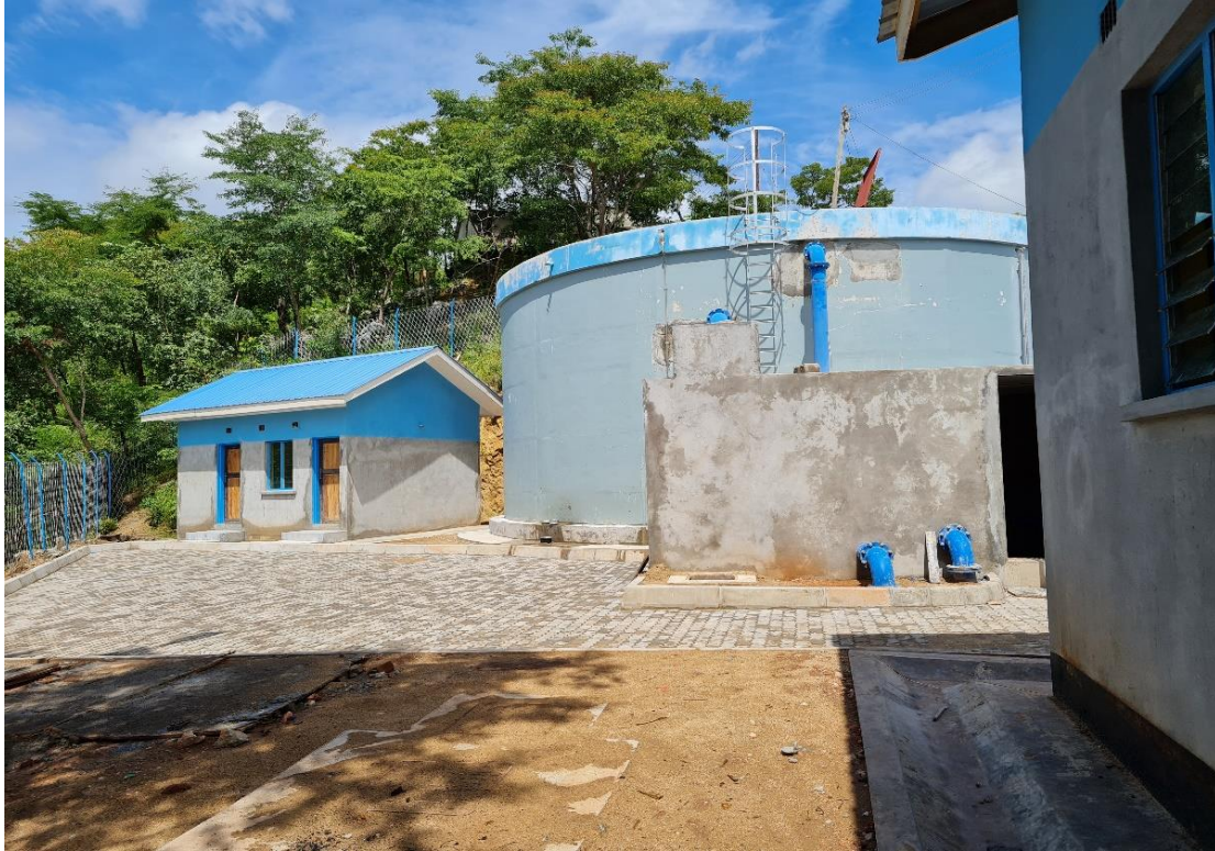
500m 3 Bwelero Tank showing tank concrete works completed.
