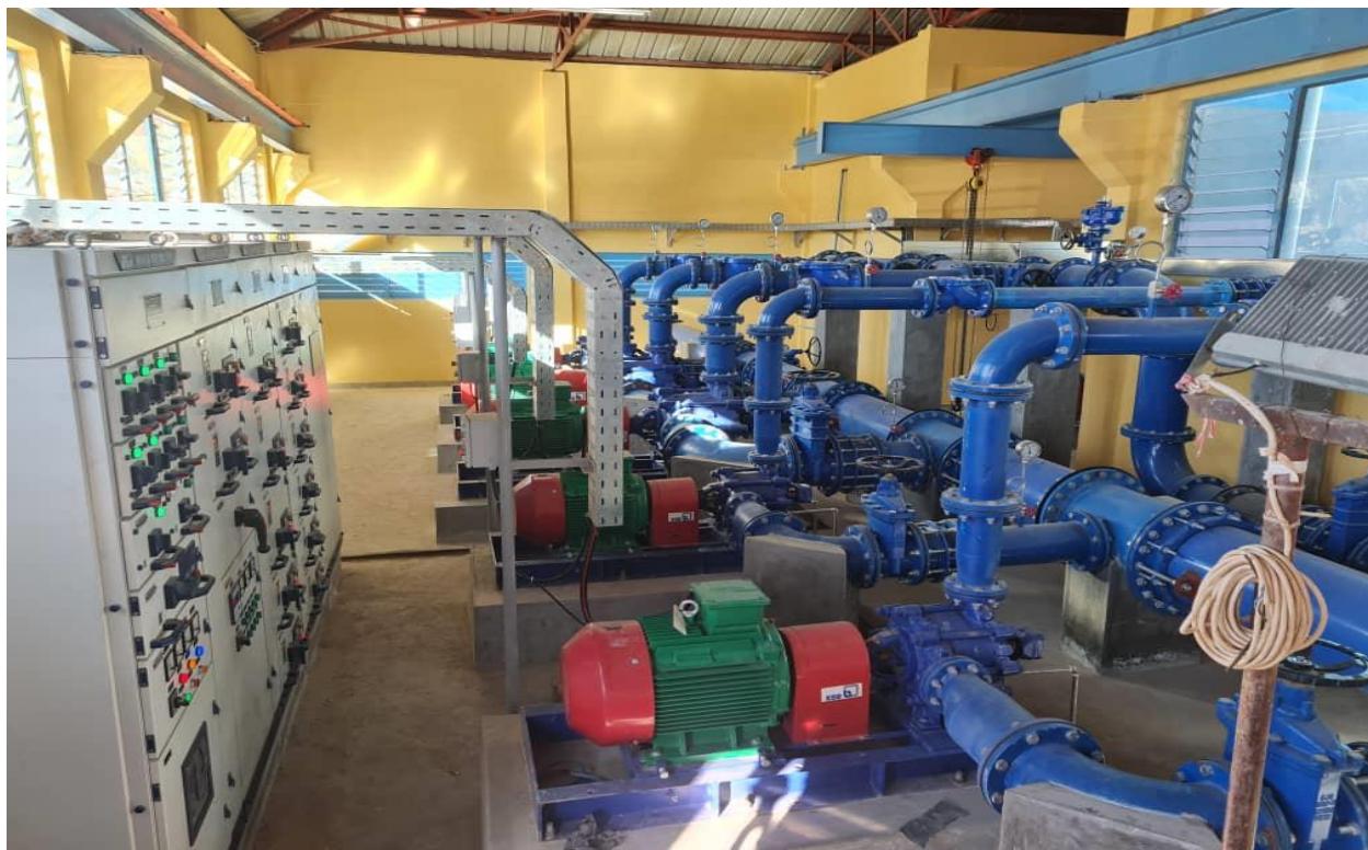
Water Treatment Plant -High Lift Pumps
